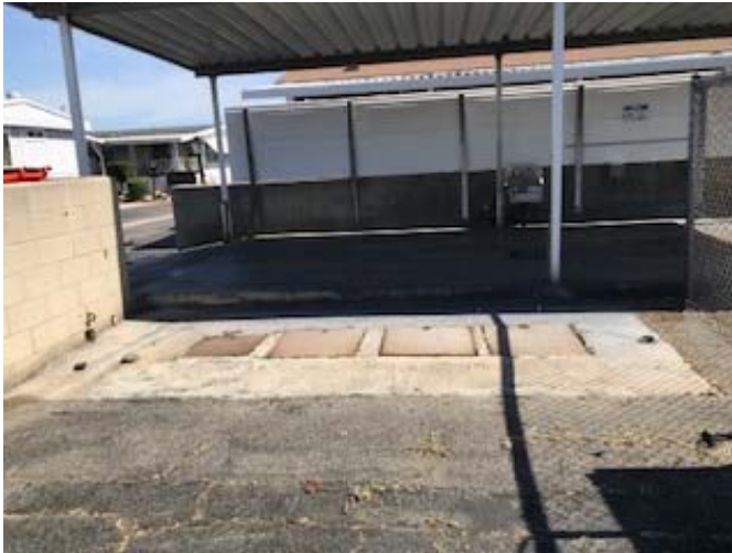
7. View of the car wash area and clarifier at the northwestern portion of the Site.
