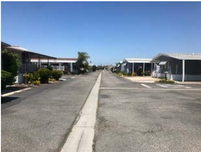
9. View north of a typical lane.
