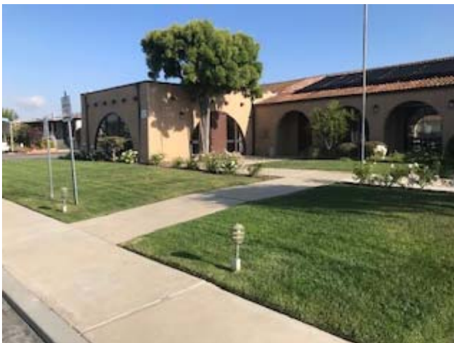
11. Northern view of the clubhouse/office.
