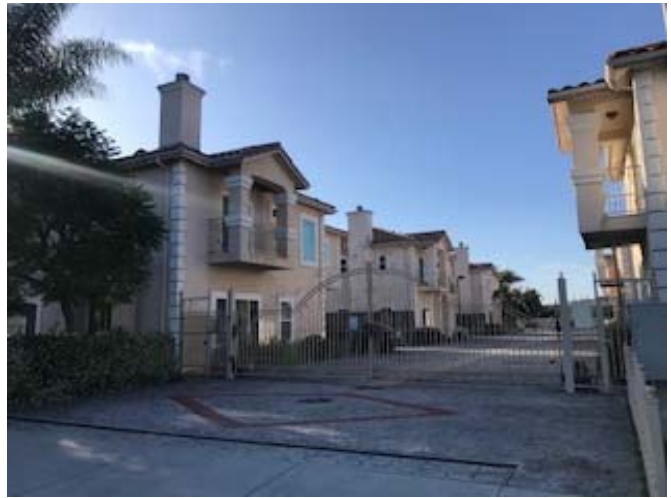
26. View of the southern adjacent residential properties.
