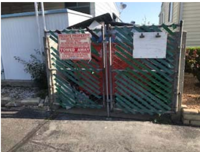
5. Typical trash enclosure.
