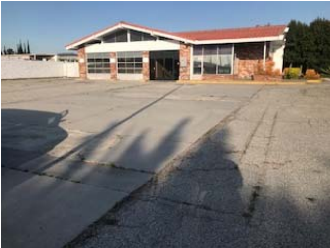
21. View of the northeastern adjacent former gas station property.
