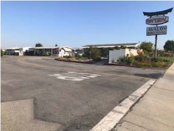
1. View northwest of the Site entrance.
